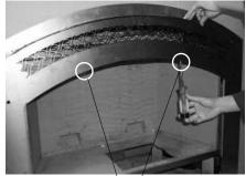
Tighten both screws to secure Arch Surround to Glass Door.
